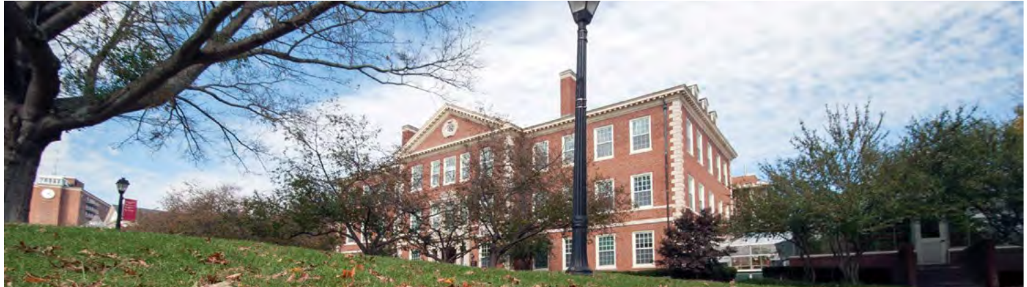
State-funded changes to Reed and Curie Halls renovate and modernize 94,840 square feet of space.
