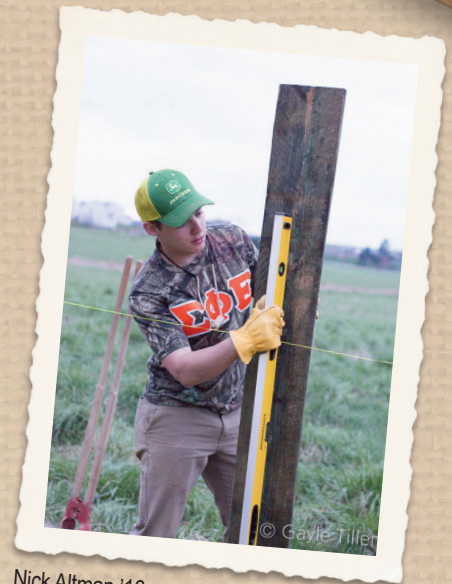
Nick Altman '16 works on repairs.
