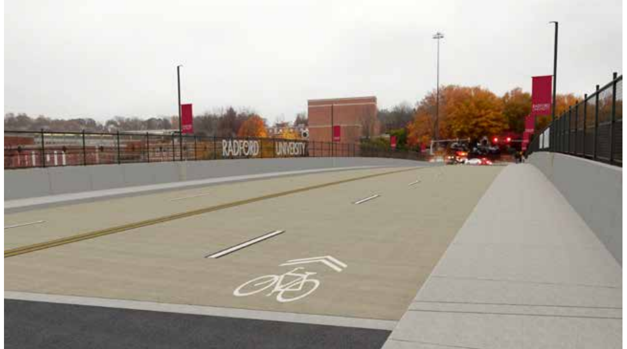
University Drive Bridge Update
